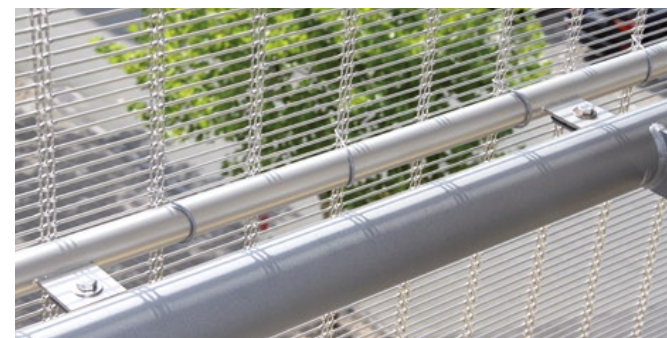
Intermediate mounting: round tube and wire connectors.
