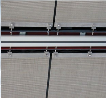
Fixed mounting system for ceiling with flat tension profiles and clevis screws.
