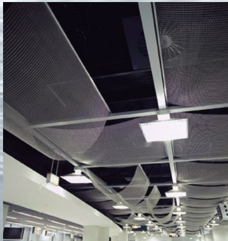
Adjustable mounting system for ceilings with sag.
