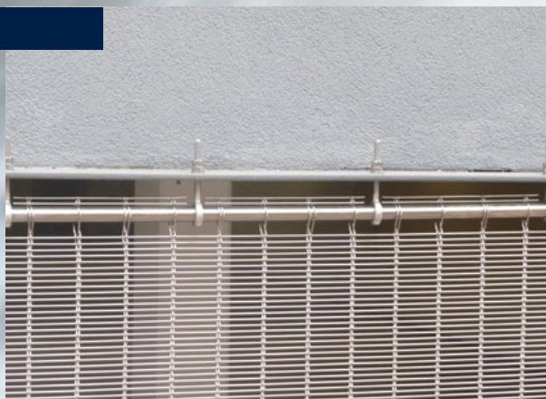
Top mounting: round bar with eyebolts.
